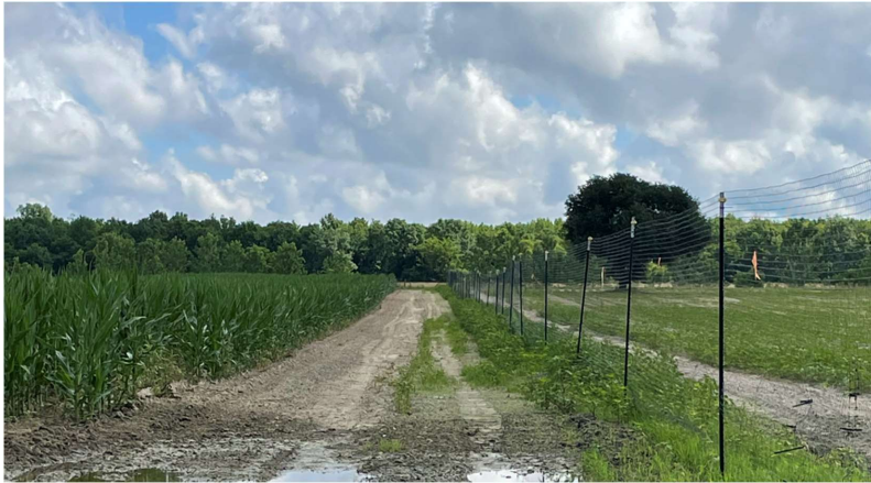
An 8 foot high polypropylene fence around a corn field. Flagging helps make the fence more visible to deer.
