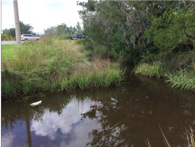
Existing culvert under Sea Island Road, to be extended for sidewalk installation.
