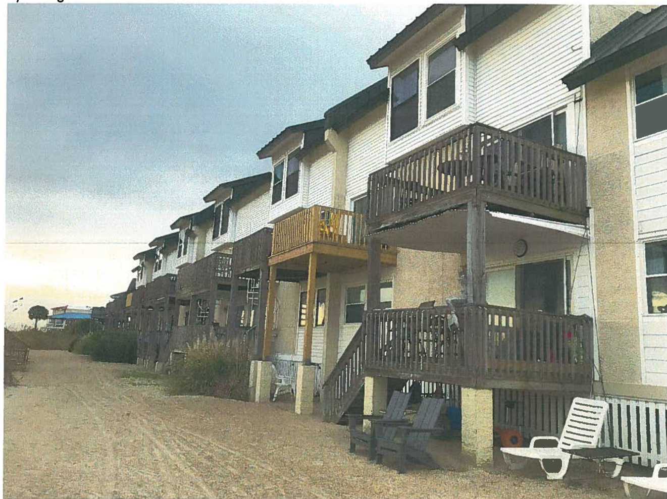
116B Butler Avenue Tybee Lights Deck Maintenance
