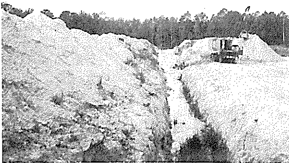
A sanitary landfill with proper cover as well as grading and drainage to prevent contamination of the water table.
