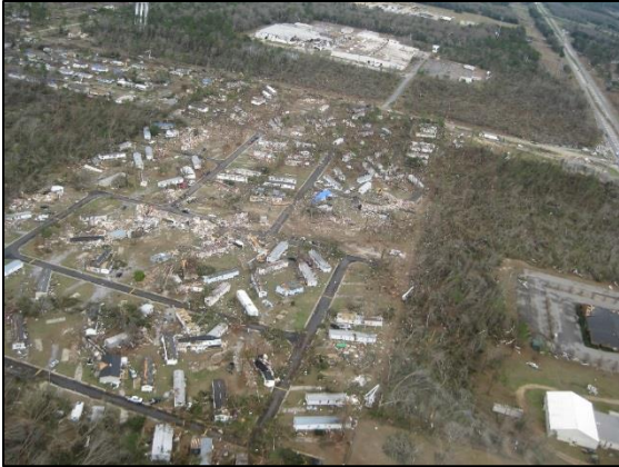
Aerial view of the Holley Drive Trailer Park in Albany destroyed by F-3 tornado on January 22 nd . Five people were killed here by the F3 tornado that traveled through Baker, Dougherty, Worth and Crisp counties.
