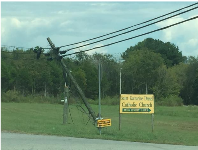
A train hit a power line which broke two power poles on Highway 11 in Dade County.
