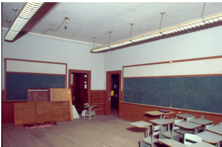
Prior to the renovation, this classroom had original blackboards and beaded wainscoting that were intact.
