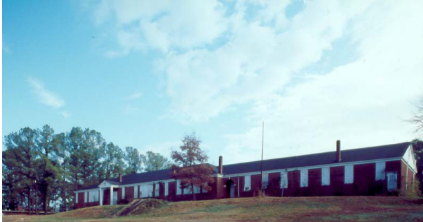
Classrooms and the auditorium were added to the north end of the building to relieve overcrowding. Photo by James R. Lockhart
