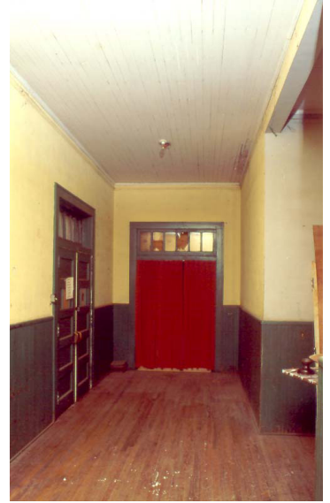
The classrooms with wood doors and transoms were saved in the preservation of the Main High School building. Photo by James R. Lockhart
