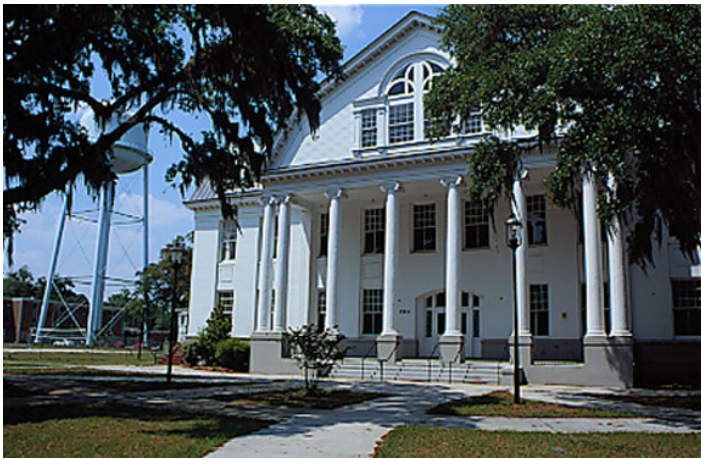
Hill Hall was completed in 1901 by students who were supervised by by trade instructors. The building materials consisted of masonry, wood and metal, and the students received proficiency certificates in the mechanical arts program that was offered at the college. Photo by Jeanne Cyriaque
