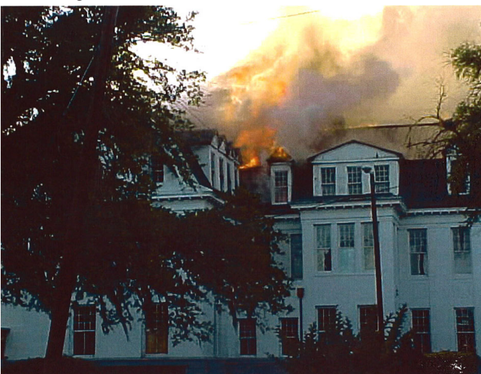
Exterior repairs including a new roof, windows and doors were completed when a fire struck the building in May 2000.
