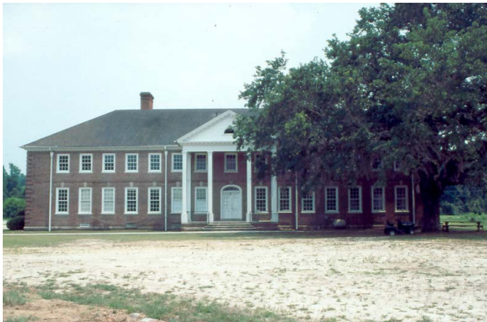
The boys' dormitory was renamed Elizabeth B. Moore Hall in honor of the first African American female president. This Georgian Revival style brick building was listed in the National Register of Historic Places on June 23, 1986. When the school closed in 1940, it became the Dorchester Cooperative Center. In the 1960s, the building provided meeting space and lodging for participants of the Citizenship Education Program. Photo by Jeanne Cyriaque
