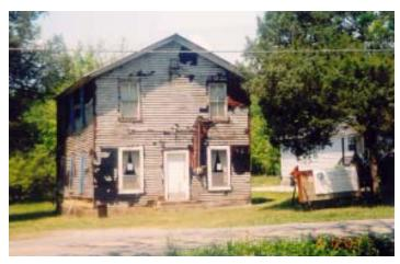
The preservation plan revealed several structural deficiencies and safetyissues. The red asphalt siding was removed and revealed the originalwood siding.Photo courtesy of WCAAHAA
