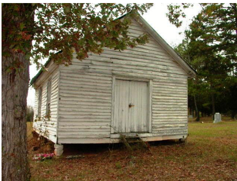
The Cherry Grove School is located next to the Cherry Grove Baptist Church and Cemetery in Wilkes County. It is a rare, one-room, wood frame building and is distinguished by its stone pier foundation.
