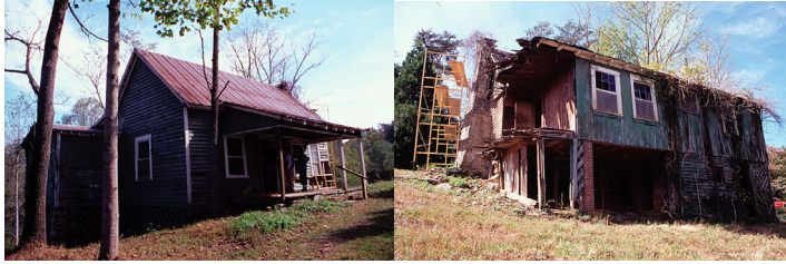
The slave cabin's original appearance was modified by adding interior rooms, windows and a front porch. These deteriorated elements were removed to restore the slave cabin to its original size. Photo by Jeanne Cyriaque
