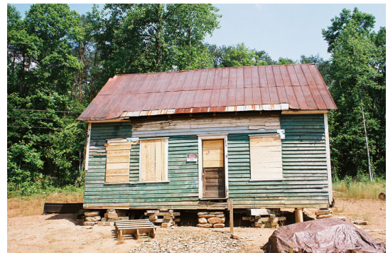
This photo shows the slave cabin resting on the original rock piers in its new home at the Nacoochee Valley African American Heritage Site & Nature Preserve. Stone mason David Vandiver will reassemble the rock chimney and hearth. Photo by Jeanne Cyriaque
