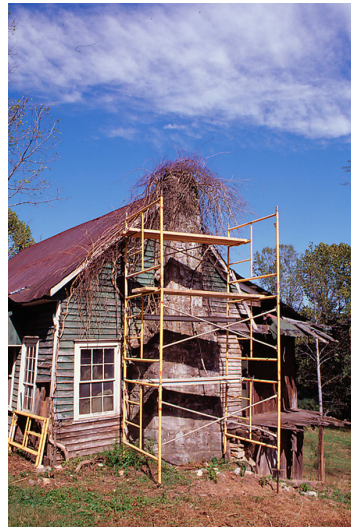
Stone mason David Vandiver stabilized the chimney that was falling into the cabin. He will reassemble the chimney to its original form.
