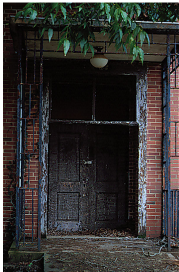
The wooden doors and arched entrance to the main hallway of the dormitory are defining features of the building. Photo by Jeanne Cyriaque
