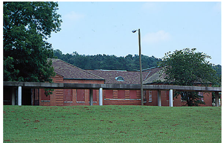
Today, a concrete walkway stands in front of the old dormitory on the Gordon Campus and provides a shelter for students. It extends to the dormitories that were added for boys and girls in the 1960s.
