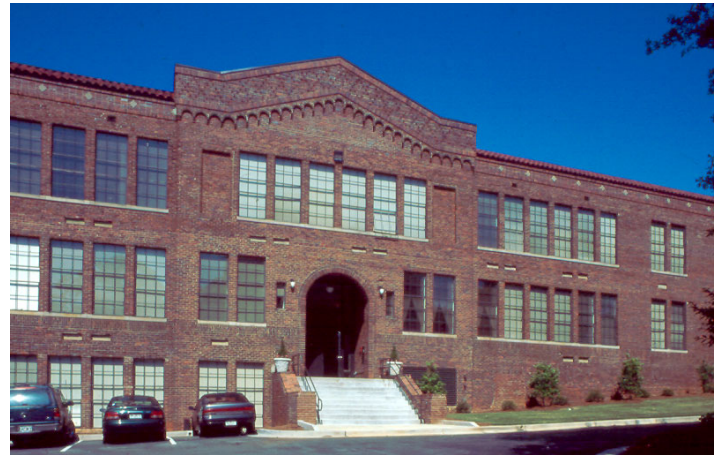
The historic Croghan School is located in the Pittsburgh Historic District. The building is adaptively used as loft apartments today and provides housing for community residents. Photo by James R. Lockhart
