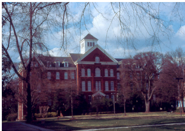
Giles Hall is a five-story, T-shaped building that is the anchor of the north end of the historic Campus Oval. The building's historic use was to provide housing and classrooms. Today, it is a multipurpose academic building.
