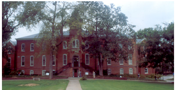
Packard Hall was named after co-founder Sophia B. Packard. It was dedicated in 1888, and provided additional classrooms, a library and dormitory space for boarding students. Today, renovations are completed, and the building is the center for student services. Photo by Jeanne Cyriaque
