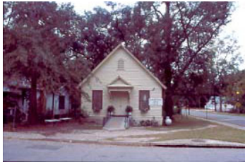
The Clay Street YMCA building is a community landmark building in Thomasville's Stevens Street Historic District. It was built circa 1890 to provide recreation services to the African American community. Today, the building functions as True Vine Church of Deliverance. It is owned by the Douglass High School Alumni Association. Photo by Jeanne Cyriaque
