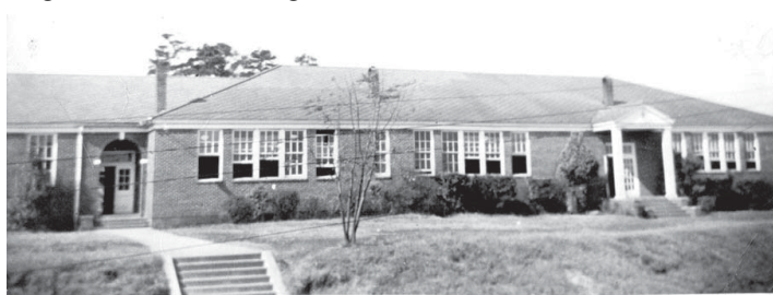
Main High School, circa 1934. The school is a one-story, stretcher-bond brick veneer structure, with a brick foundation and eight brick chimneys. It originally contained four classrooms, two restrooms, and a small office. By 1938, two additional classrooms and an auditorium were constructed, designed by Atlanta architect, Odis Clay Poundstone. Photo courtesy of Rufus N. Turner Jr.
