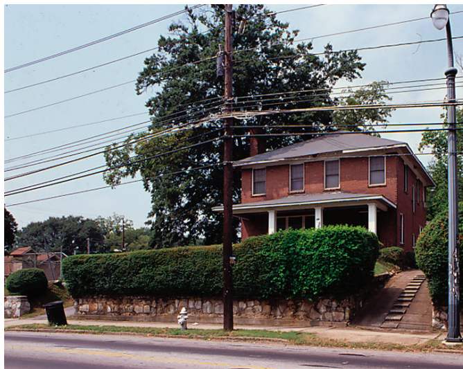
The home of Brailsford Reese Brazeal was listed in the National Register of Historic Places on April 8, 2005. Photo by James R. Lockhart
