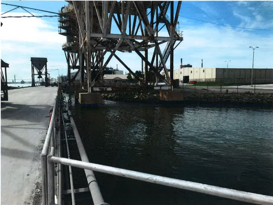
Photograph 1: Upstream End of Existing Facility. Photograph Shows the Location of New Proposed Decking on the Bottom of the Photograph and Proposed Conveyor Support Platforms on the Inside of the Existing Dock.
