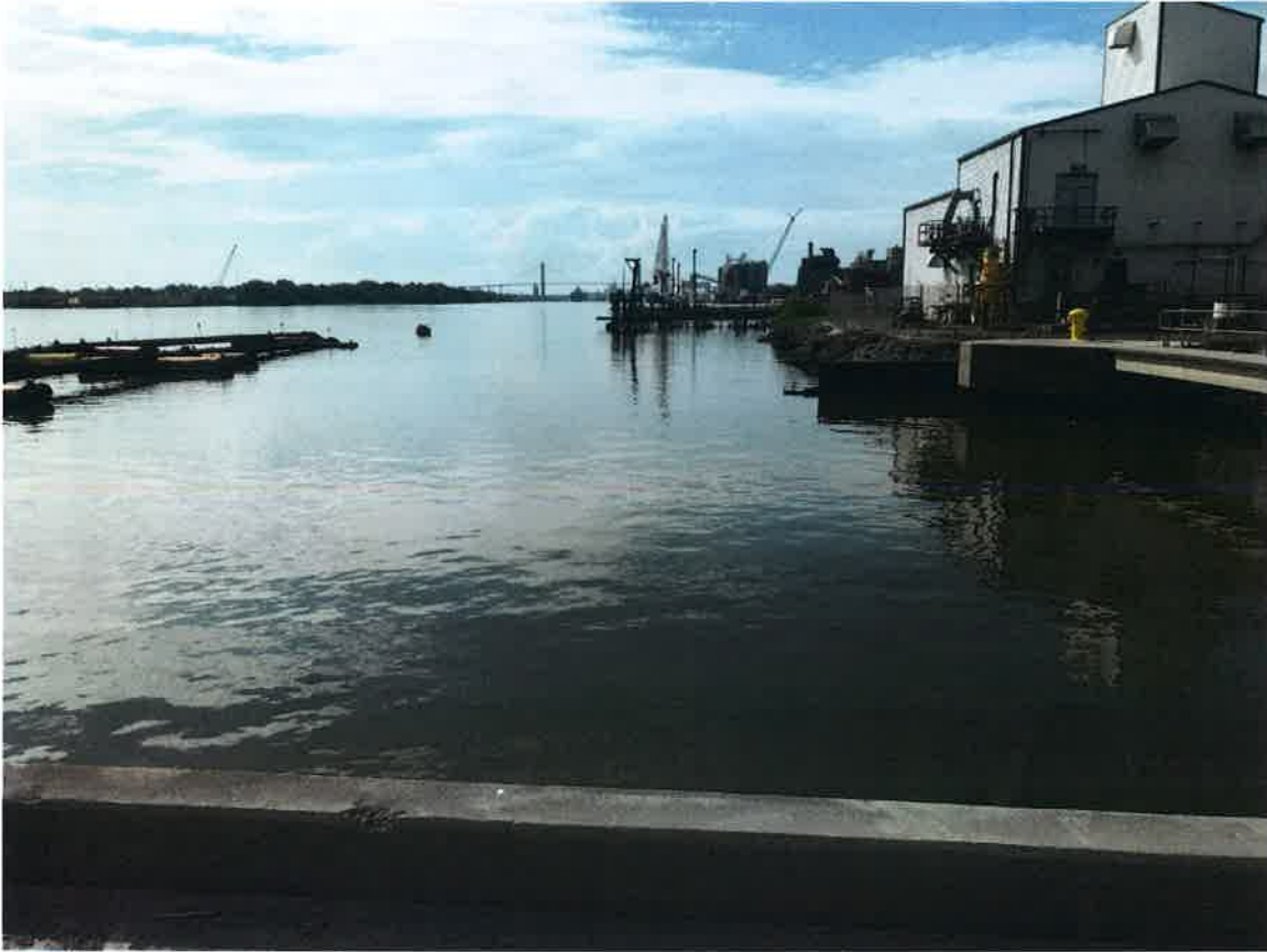
Photograph 2: Downstream View. Photograph Shows the Location of Proposed Deck Extension on the Downstream Side of the Dock. The Walkway on the Right Side will be Removed. The Mooring Dolphin will Remain.
