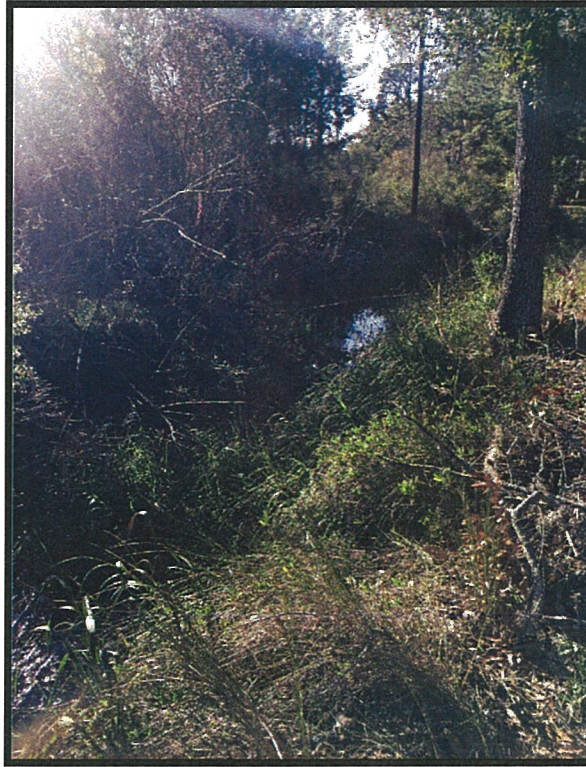
Photo 5: Tidal ditch, facing upstream from pedestrian bridge crossing
