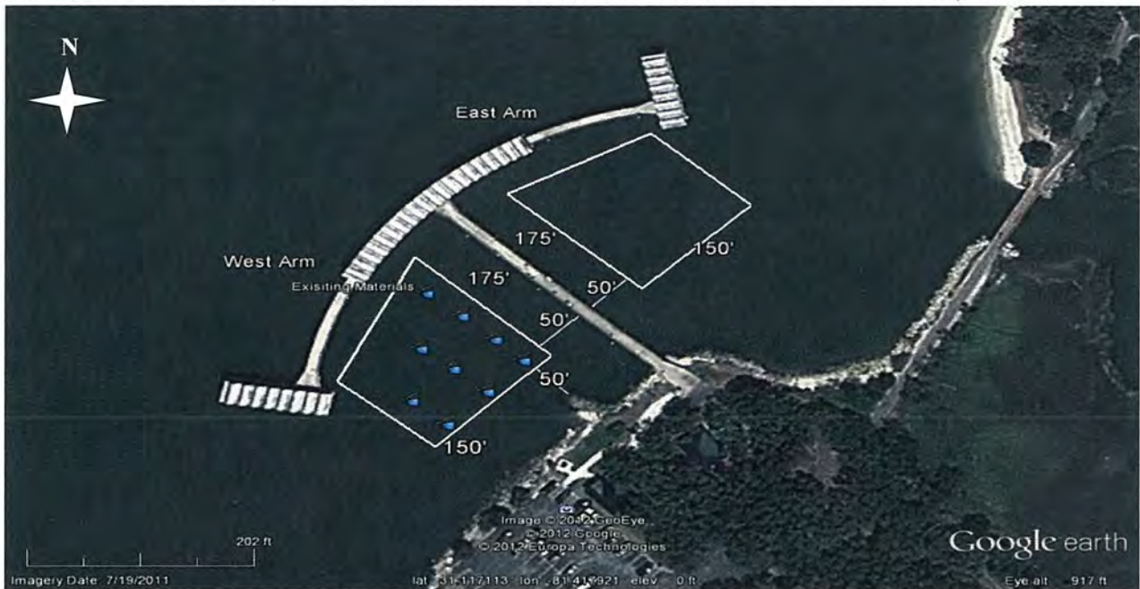
Figure 2. Aerial Photograph of the Jekyll Pier Inshore Artificial Reef Site. Existing materials/footprint (175' x 150') on the west arm of the pier and footprint (175' x 150') for the east arm of the pier.
