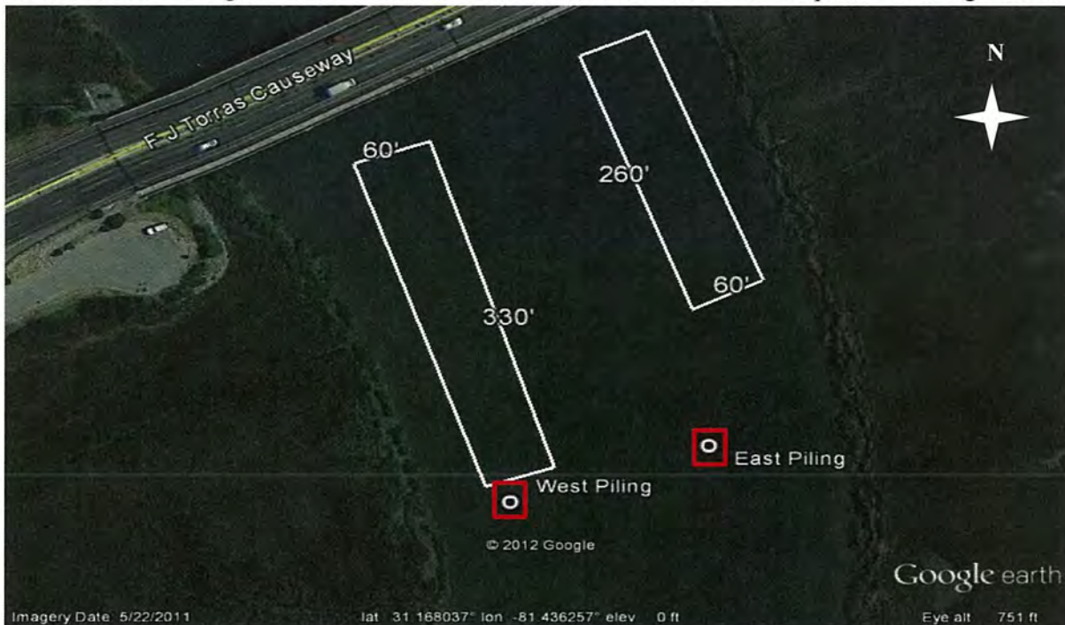
Figure 2. Aerial Photograph shown with existing pilings, materials, and footprint (West Bank: 330' x 60', East Bank: 260' x 60'). Pilings outlined in red are for navigational purposes.
