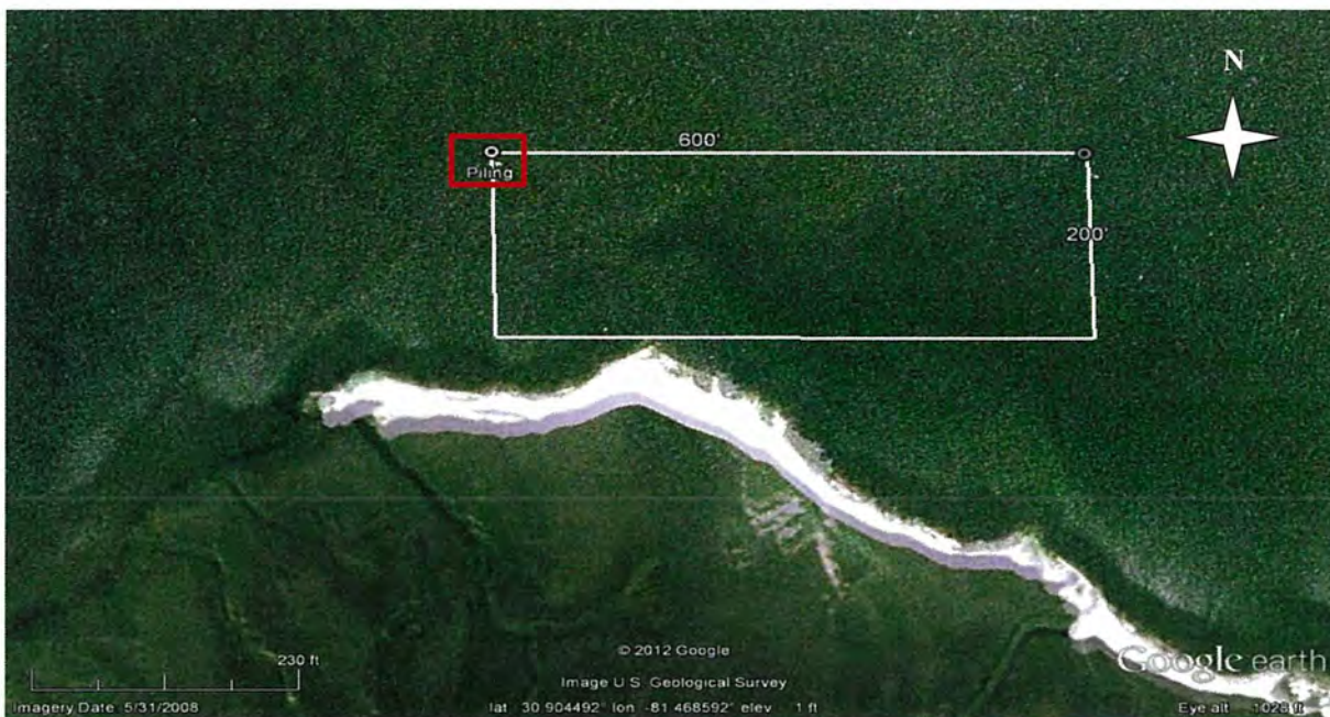
Figure 2. Reef Site Aerial Photograph shown with existing pilings, materials, and footprint (600' x 200'). For navigational purposes the southernmost piling is outlined in red.
