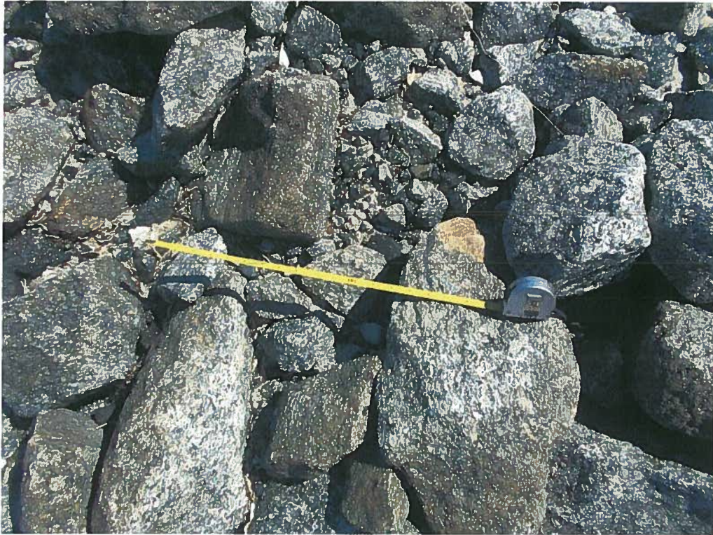
Distribution of existing stone near north limit of revetment
