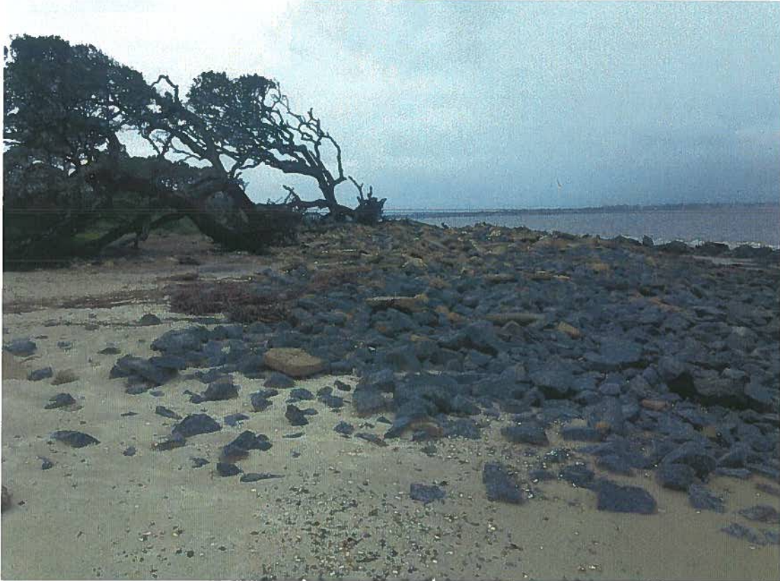
Photo of widely scattered small stone near north project limit (north of Villas by the Sea, south end of Driftwood Beach). Photo taken at low tide, 8/21/17
