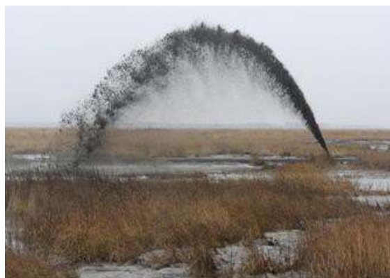
Figure 2. TLP of dredged material using high pressure hydraulic spray during restoration of marshland in the Blackwater National Wildlife Refuge, Maryland.
