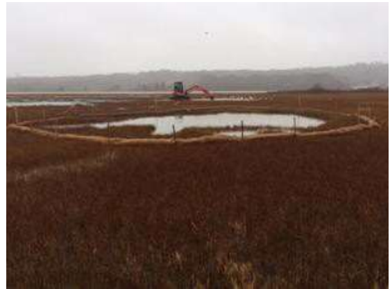
Figure 3. Example of the use of bagged oyster shells as containment for TLP of dredged sediment on marshland in the John H. Chafee National Wildlife Refuge, RI.
