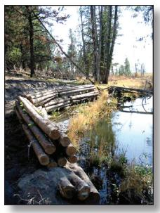
Figure 4.5.11b Stream Channel After Log Revetment Photo Courtesy of: rrnw.org
