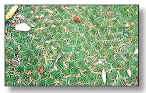
Figure 4.5.4c Hexagonal Cells Filled with Turf for Bank Reinforccement Photo Courtesy of: Pavingexpert.com
