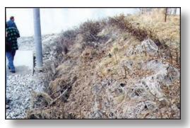
Figure 4.5.3b Biodegrading Coconut Mat Along Bank
