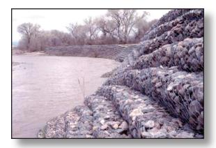
Figure 4.5.9a Tiered Installation of Rock Gabions Photo Courtesy Of: Tostreams.org
