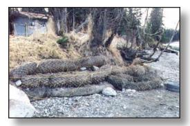
Figure 4.5.3d Installation of Straw and Coir Log Along Stream Bank at Low Tide Photo Courtesy of: Tellusnews.com
