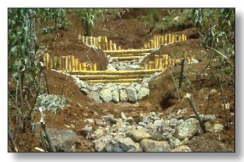
Figure 4.5.12a Wooden Weirs Stream Channel Photo Courtesy of: Zeitlow.com
