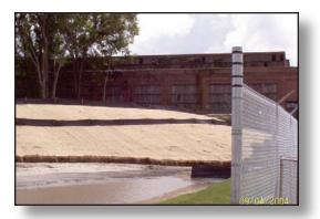
Figure 4.5.3c Jute Mesh Covering Slope Photo Courtesy of: Matt Renault
