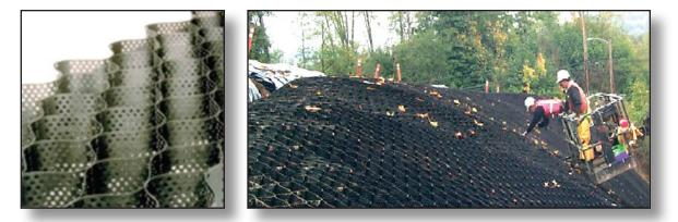
Figure 4.5.11c GeoWeb Material Photo Courtesy of: Geocheminc.com
