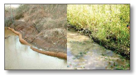
4.5.2a Stream Bank Before and After Stabilization with Vegetation Photo Courtesy of: Nagreen.com
