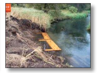
Figure 4.5.11f Fish Lunker Structure Photo Courtesy of: fmr.org
