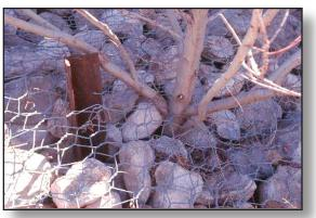
Figure 4.5.9d Willow Tree Growing from Gabion Photo Courtesy Of: Tostreams.org
