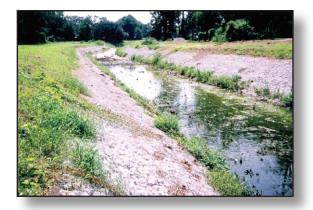
Figure 4.5.9c Vegetation Taking Hold on Rock Gabion
