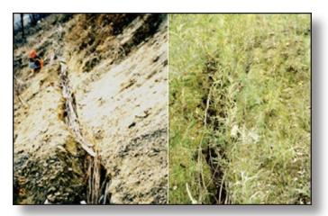
Figure 4.5.8a Brush Trench with Willow Cuttings During and After Construction
