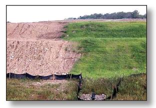
Figure 4.2.1a Vegetated Slope vs. Non-vegetated Slope with Rills and Gullies
