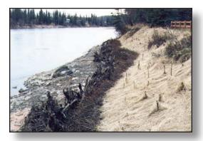
Figure 4.5.3a Coconut Mat on Stream Bank Photo Courtesy of: Chere Peterson
