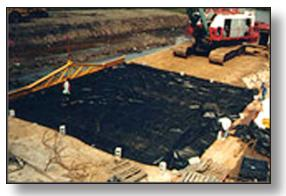
Figure 4.5.4a Filter Fabric Applied to a Moderate Slope Photo Courtesy of: US Fabrics, Inc.
