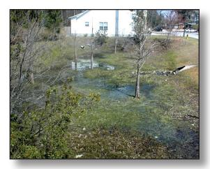
Figure 3.3.5e Infiltration Basin After Rain Event
