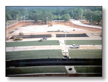
Non-structural systems such as turf, reinforced with synthetic grids, can also be used as paving in some instances. Local materials such as crushed shell can be employed as can cobbles or gravel in some applications. Gravel, sand and even mulch can be used to pave pedestrian pathways, depending on usage requirements.
