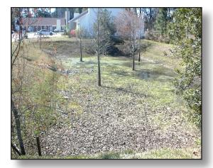
Figure 3.3.5f Dry Infiltration Basin 12 Hours After Rain Event
