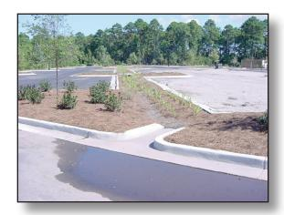
Figure 3.3.4b Bioretention Swales with Curb Cut
