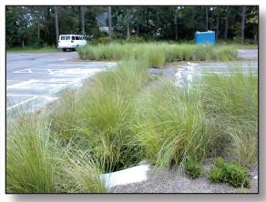
Figure 3.3.4c Bioretention Swales Using Wheelstops
