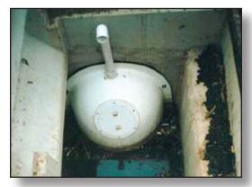
Figure 3.3.9d Snout Structure in Place Photo Courtesy of: Bestmp.com
