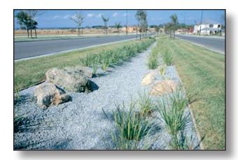
Figure 3.3.5a Infiltration Trench in Highway Median Photo Courtesy of: Dot.state.ohi.us
